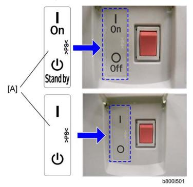
19. Attach the on/standby decal [A] to the left-hand side of the main power switch.
