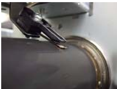
Correct position of the thermistor
